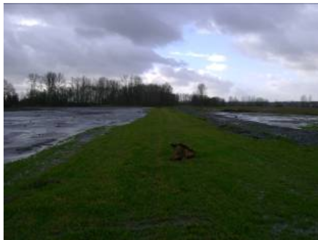
This is another shot of the newly completed dike. The farm is to the right and the area to be restored for salmon to the left. The Nooksack River lies beyond the line of trees in the distance.
