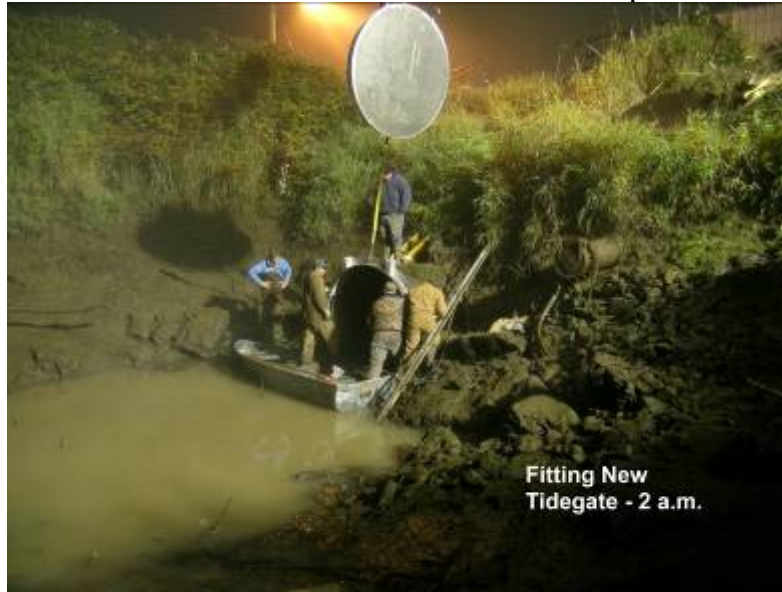
Workers installing the new, aluminum tide gate.
