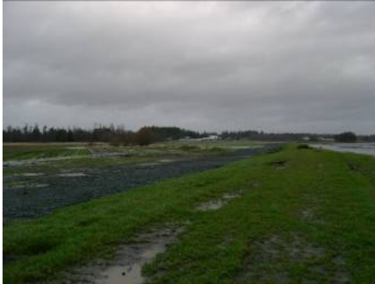
This shot, taken in December 2006, shows the good condition of the new Bertrand Creek dike shortly after the November flood. One of the protected farms lies to the left, with Bertrand Creek shown to the right.
