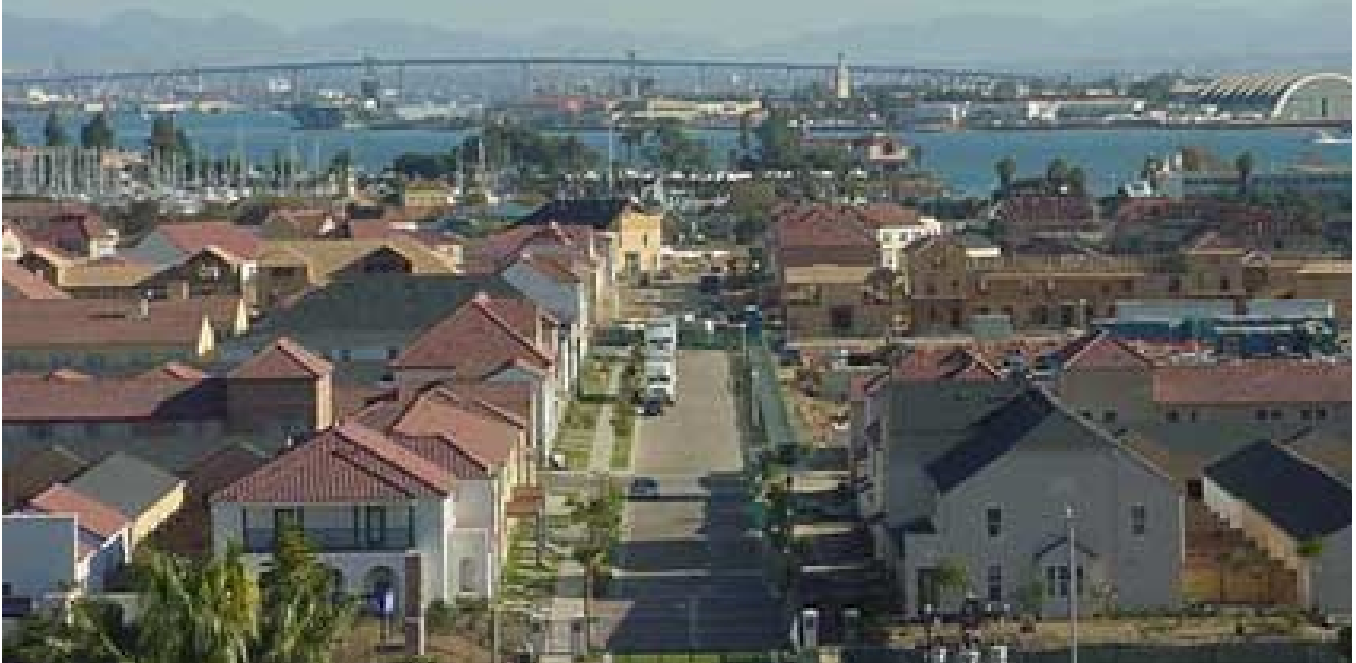
A view of the Village with construction nearly completed.
