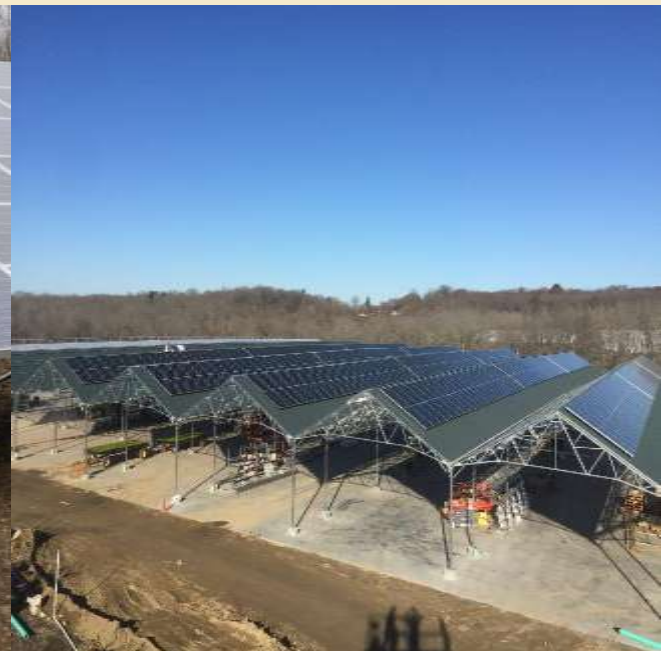
Prides Corner Farm in Lebanon, CT installing 240 kW solar system on a newly constructed greenhouse structure.
