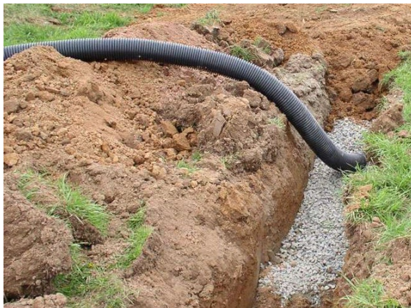
2:90-2.18 Underground drainage systems
