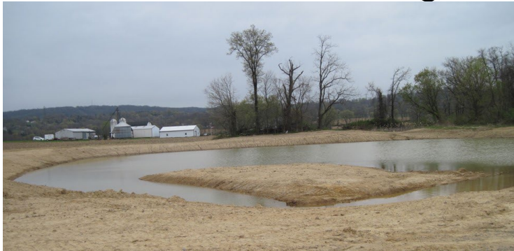
2:90-2.14 Water impoundment reservoirs
